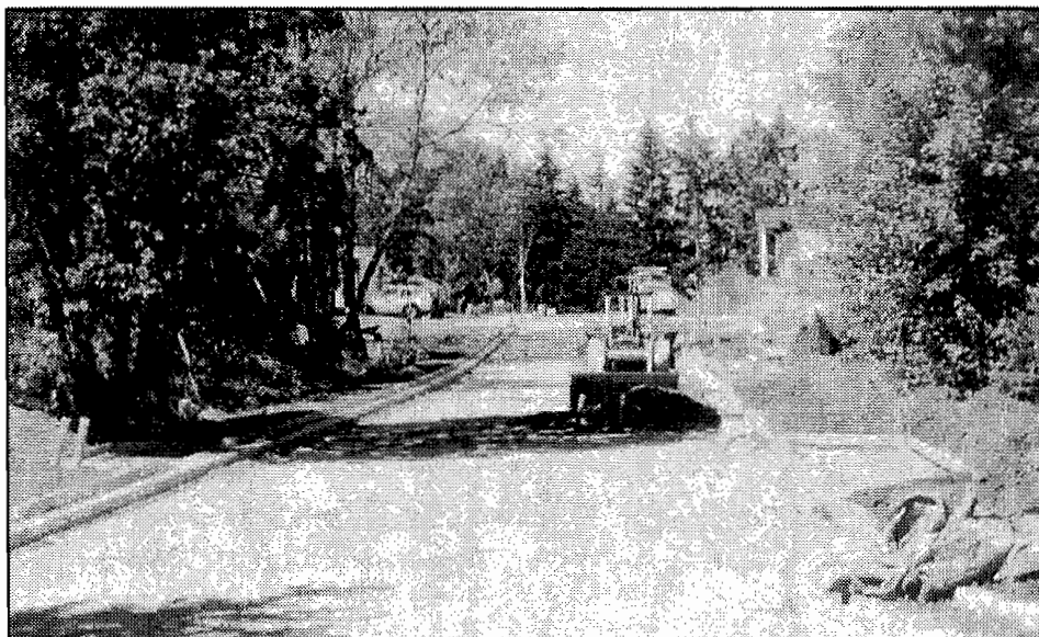
Figure 2. Road construction on Lambert Street South in West Eugene.
